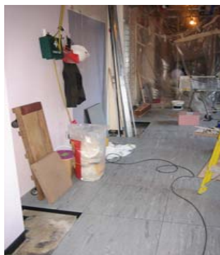
New suspended floor
